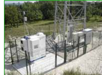
France – Bouygues Telecom
