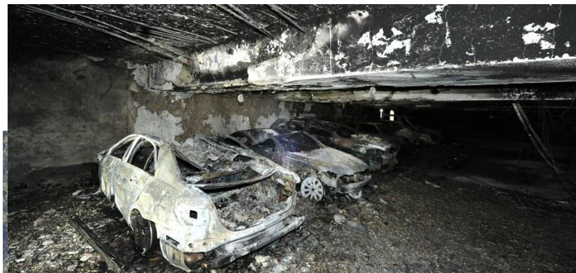
2012 - Incendie de parking souterrain place Vendôme
