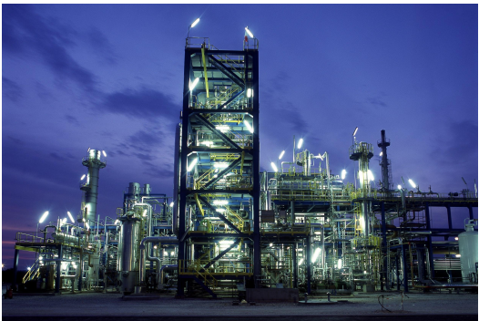
Chemicals & Petroleum refining
