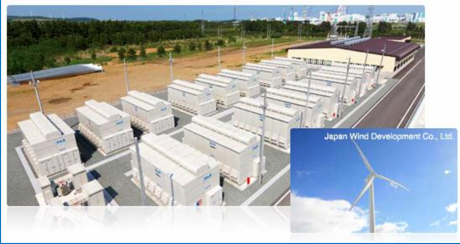
34 MW NAS alongside 51 MW Wind Farm
