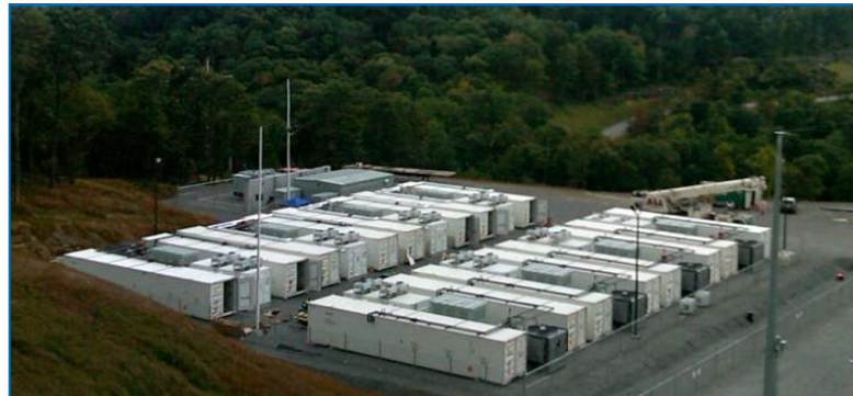
32 MW lithium-ion battery for a 98 MW wind farm (US)
