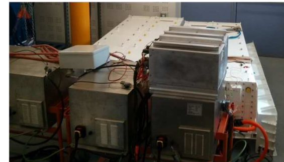
CEA Battery Modules
