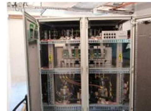
250kW charging station
