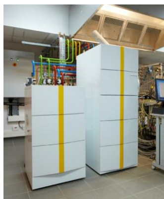
CERAMIS POWER DE DIETRICH (SOFC)
